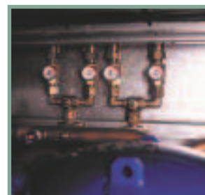
Dual pressure relief valve
